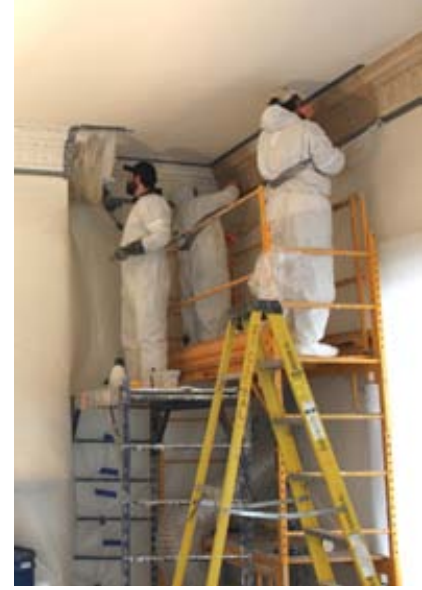
Removal of layers of paint in the Dining Room revealed that older portions of the entablature in the Dining Room were within the bow of the room and around the chimney box
