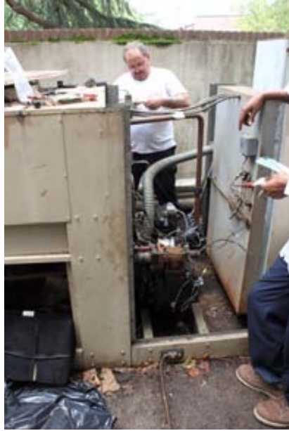
Repair of the air conditioning compressor, damaged by lightning storms this summer
